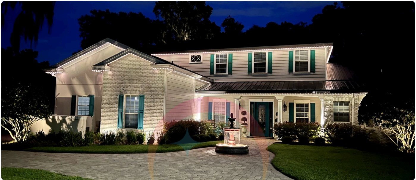
One connected platform, one app: roofline track, facade wash, and landscape lighting running together on a single Brighter Nights installation — warm white, downward beam, zero visible hardware.
