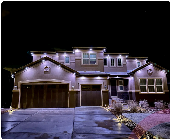
Architectural downlight pattern. Individual pixels spaced like recessed can lights; the strip between them is completely dark and invisible.
